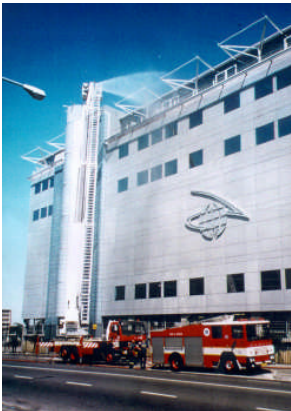
Vodacom Building South Africa
