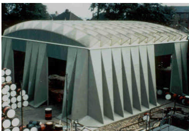
Modular Stores Building Wollaston
